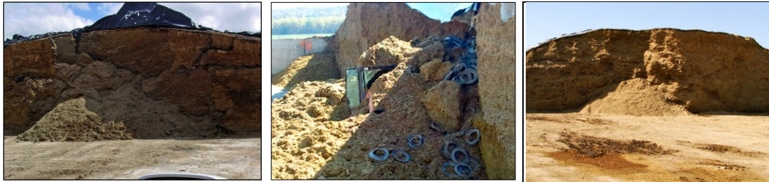
Figure 3. The photos of the two bunker silos (left and center) and pile (right) were taken minutes after the avalanches occurred. The person operating the payloader was not seriously injured.
